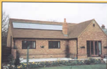
Domestic hot water and central heating (winter) and swimming pool heating (summer). United Kingdom, 120 Tubes
